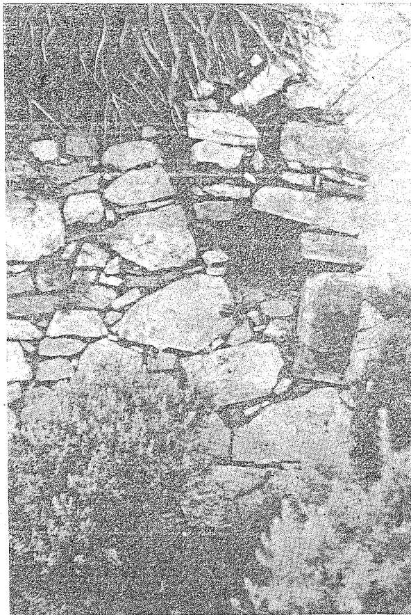
Fig. 8. Site AC-63. A corner of the wall around section A
