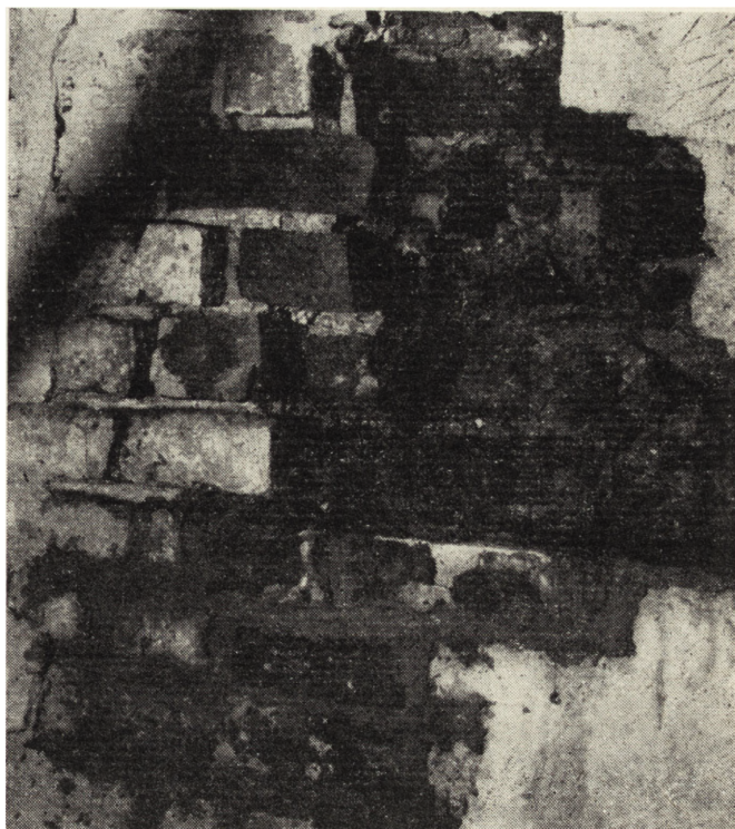
7. Lublin, castle chapel of Holy Trinity, northern wall of the presbytery — preparing of the flush from liquid mortar with hydraulic properties
