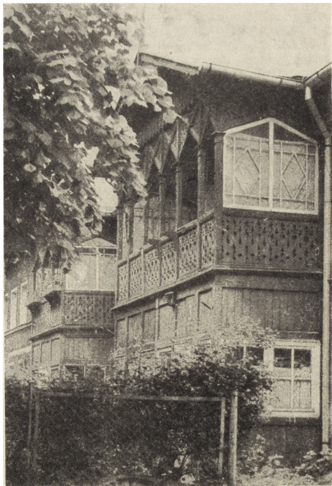
5. Gdańsk-Wrzeszcz, 3 Matki Polki street, an example of a wooden veranda — loggia in the upper floor; this is the look some of Sopot verandas-loggias might have had at the end of the 19th century before they were later glassed
