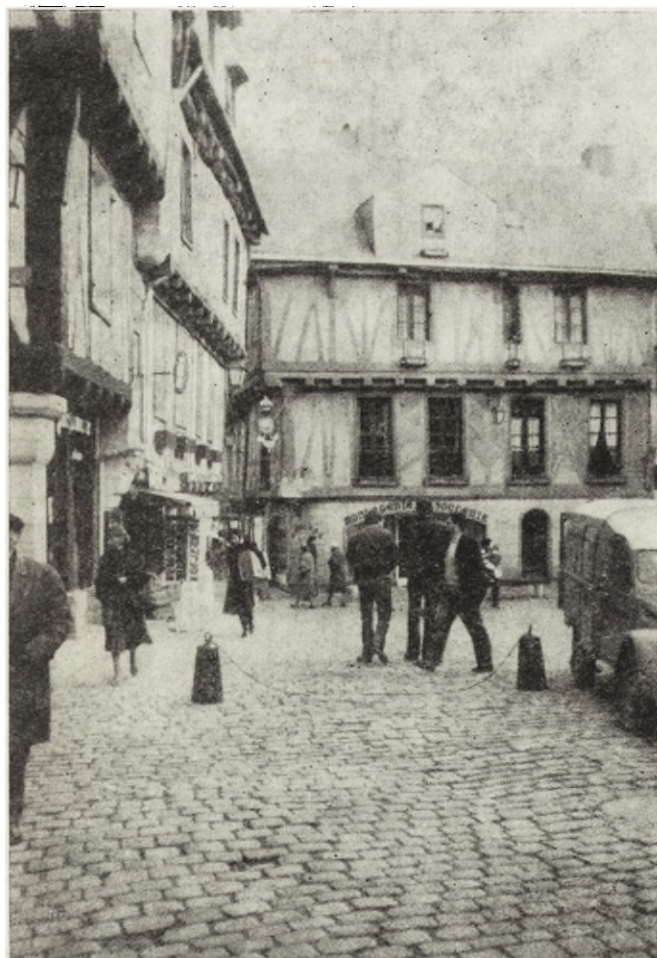
6. 7. 8. Vannes (France), details of the renewed centre
