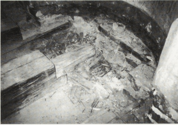
7. Skorodowane belki stropowe między parterem a piętrem pałacu 7. Corroded ceiling beams between the palace ground floor and storey
