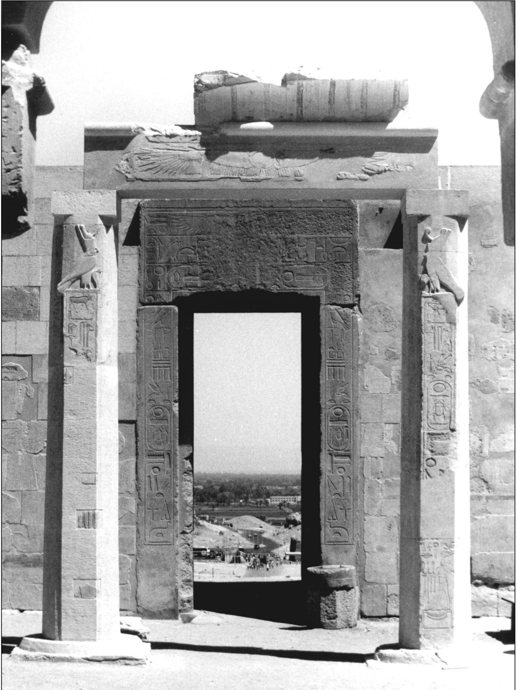
Fig. 4. Architrave restored on the main axis of the Upper Court (Photo W. Jerke)
