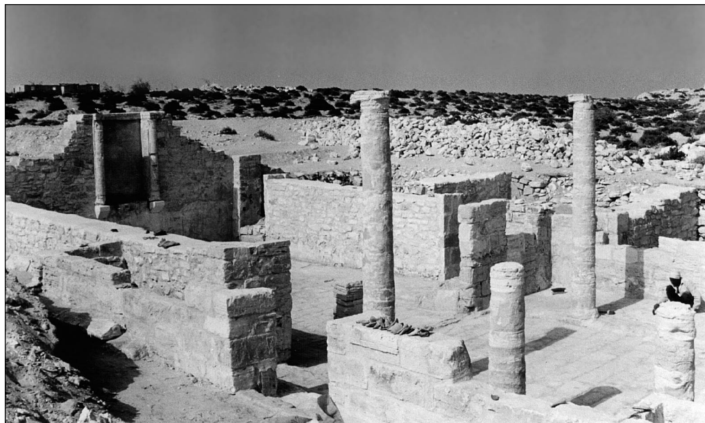
Fig. 4. House H 10. Portico courtyard and room 2 with relics of niche after restoration. View from the northeast (Photo S. Medeksza)
