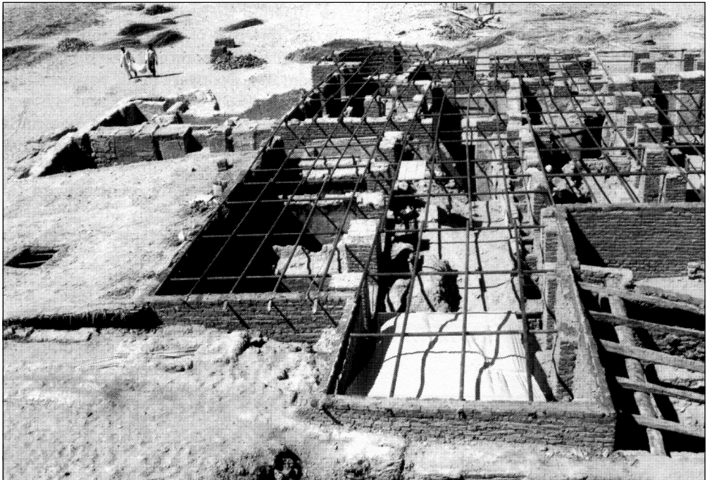
Fig. 9. Western Annex in 1998. Work on the roofing of the complex (Photo W. Chmiel)
