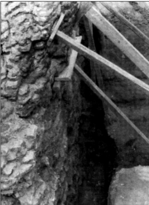
Fig. 2. Cisterns. Western wall of the corridor before restoration (Photo W. Kolqataj)
