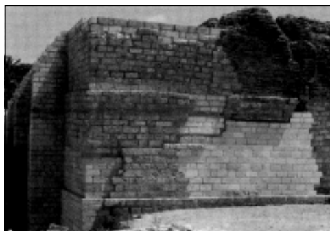
Fig. 9. Cisterns. Northeastern corner after restoration (Photo W. Kołtąj)
