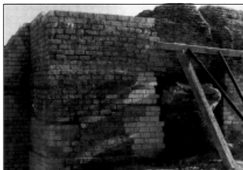
Fig. 8. Cisterns. Northeastern corner before restoration (Photo W. Kołtąj)
