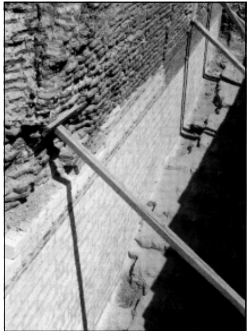
Fig. 3. Cisterns. Western wall of the corridor after restoration (Photo W. Kolqataj)
