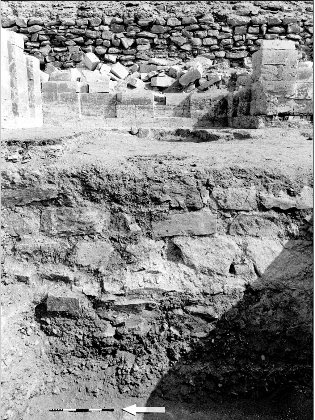
Fig. 8. Western face of the substructure supporting the enclosure wall of the complex of Netjerikhet. View from the west (Photo M. Jawornicki)
