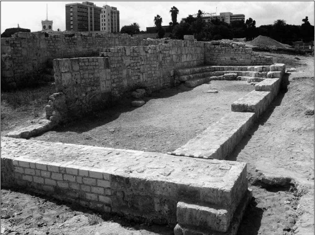
Fig. 11. Area AW. Northern auditorium (no. 2), view after restoration (Photo G. Majcherek)
