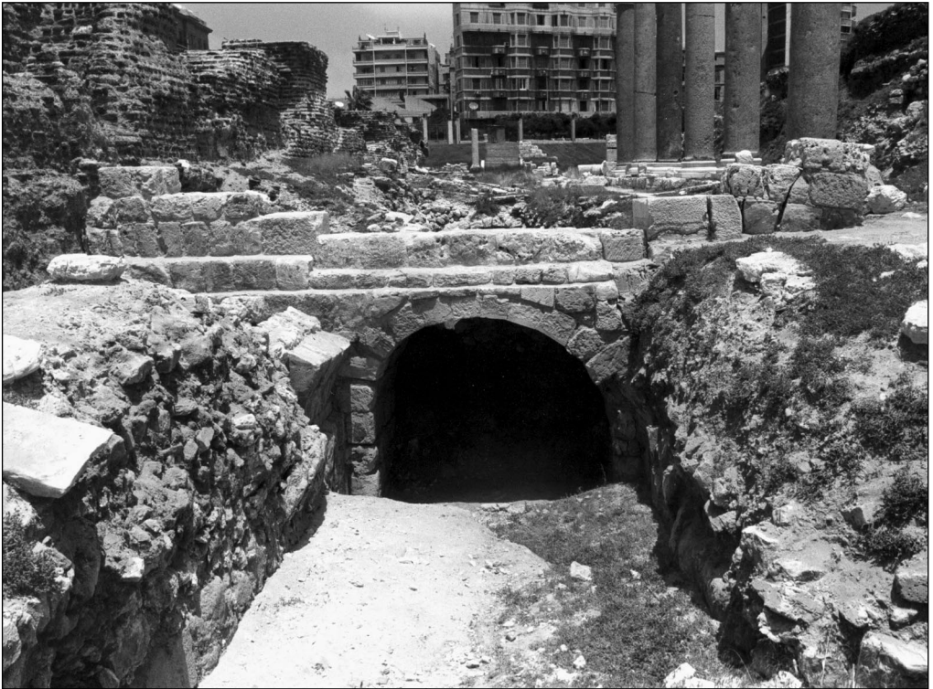
Fig. 12. Bath complex. Restored arch of the underground service passage supporting the western gateway to the baths, view after restoration (Photo G. Majcherek)
