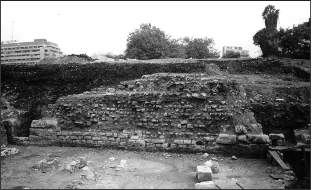
Fig. 8. Theater Portico. The back wall in sector L, view prior to restoration (Photo G. Majcherek)
