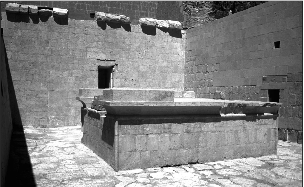
Fig. 6. The northwestern corner of the Solar Court after restoration (Photo M. Barwik)
