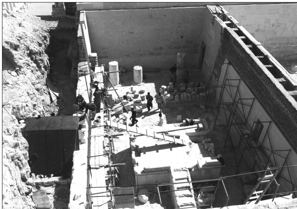
Fig. 2. Work on the construction of the north wall of the Solar Court and concrete ceiling above the Upper Chapel of Anubis (Photo M. Jawornicki)
