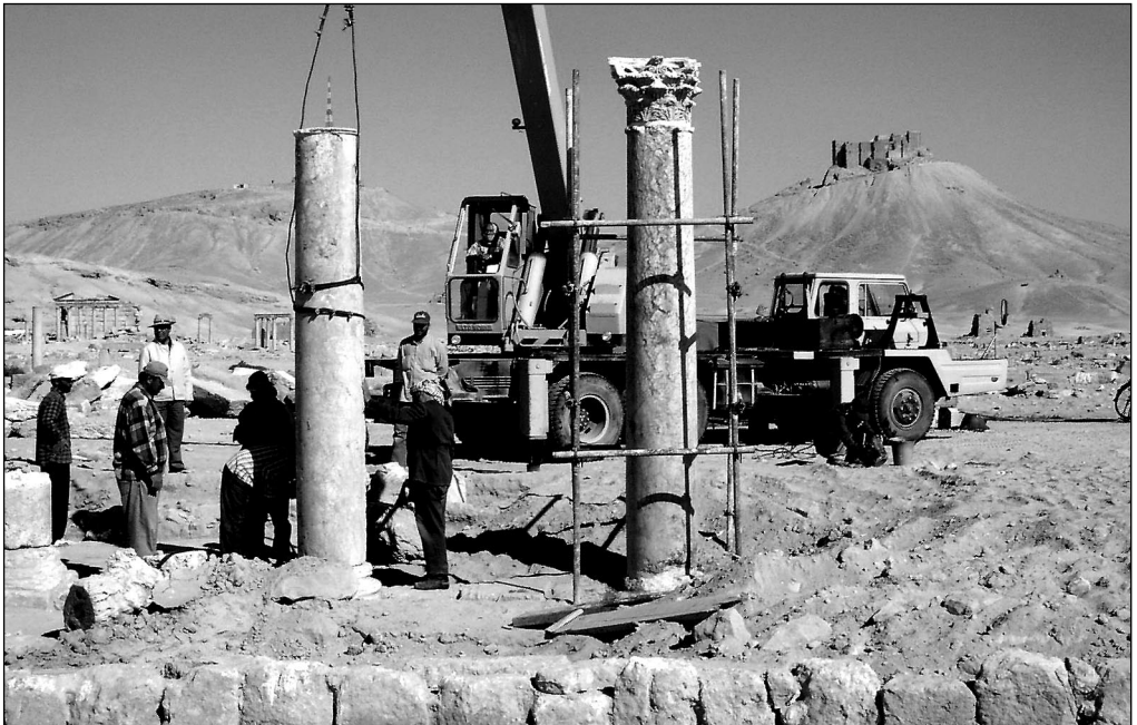
Fig. 5. Raising of the columns in the atrium of Basilica III (Photo M. Gawlikowski)
