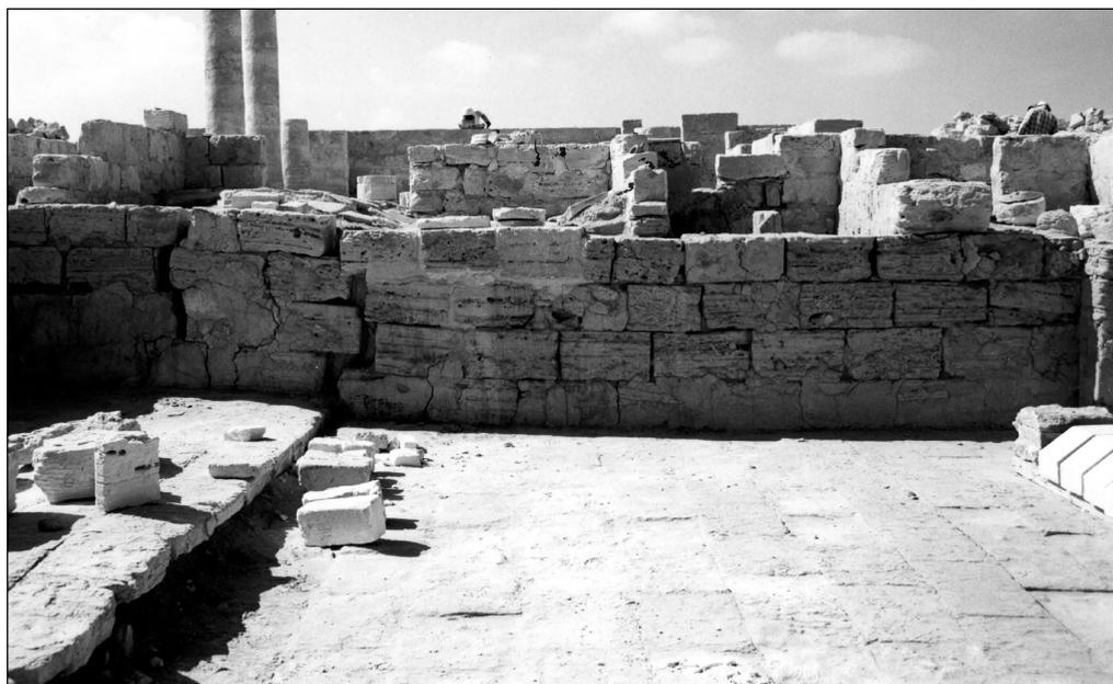
*Fig. 5a. Hall H 21 "N". Before conservation. Close-up view from the north of the cracked south wall and displaced pavement (Photo S. Medeksza)*
