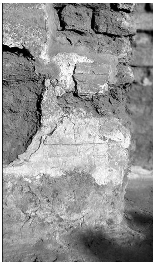
Fig. 4. Fragmentarily preserved stucco decoration on the second coating of plaster in the western arm (Photo D. Zielińska)
