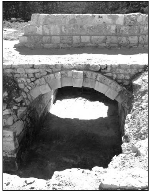
Fig. 8. Restored vault in the southern passage of the bath, looking south (Photo G. Majcherek)
