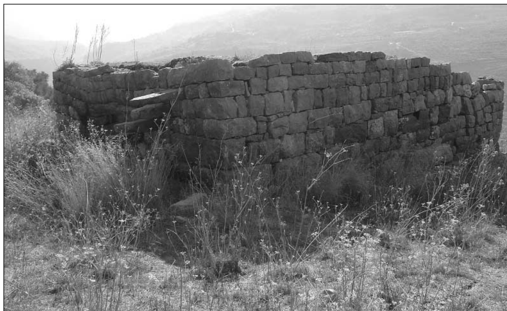
Fig. 2. Site 13, view from the northeast (Photo K. Jakubiak)
