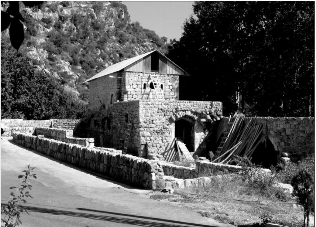
Fig. 1. The Church of Mar Sarkis in Kaftoun, state in 2004 (Photo T. Waliszewski)
