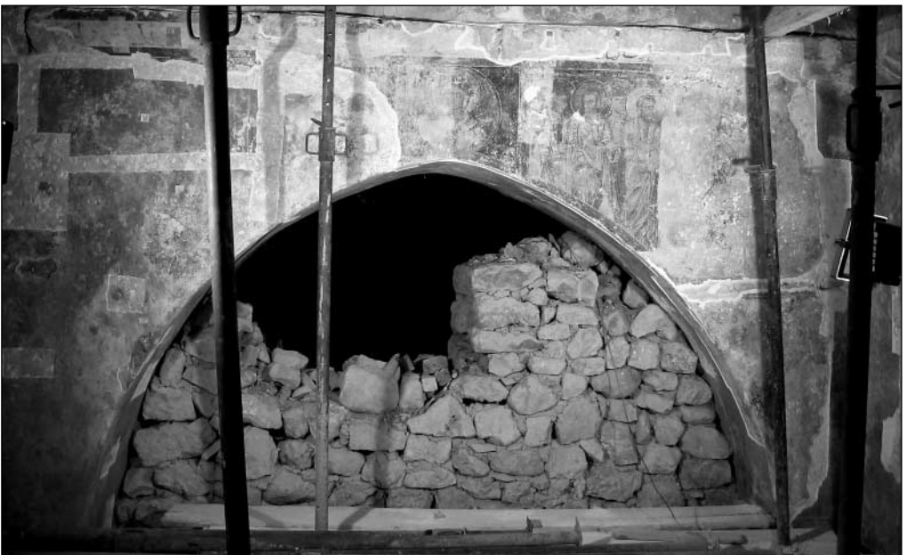
Fig. 3. North wall of the nave with uncovered traces of murals, state during conservation in 2004 (Photo A. Karolczak)
