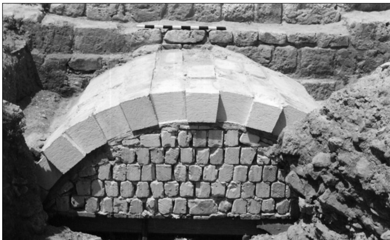
Fig. 10. Vault next to the western gate after restoration (Photo G. Majcherek)
