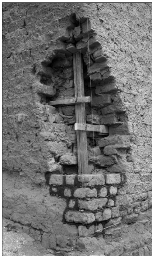
Fig. 8. Tower B during the restoration of the corner, viewed from the south (Photo T. Górecki)
