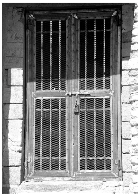
Fig. 29. Western entrance to the building of the Mosque with new mesh-net door (Photo W. Godlewski, PCMA archivess)
