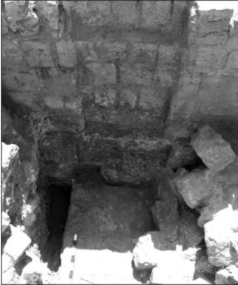
Fig. 9. Abutment of the east–west wall and the portico back wall (Photo A. Smilgin)
