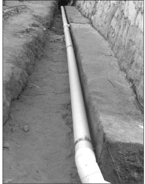
Fig. 10. Consolidated foundations and rainwater drainage of the east wall of the mosaic shelter (Photo J. Brochocki)
