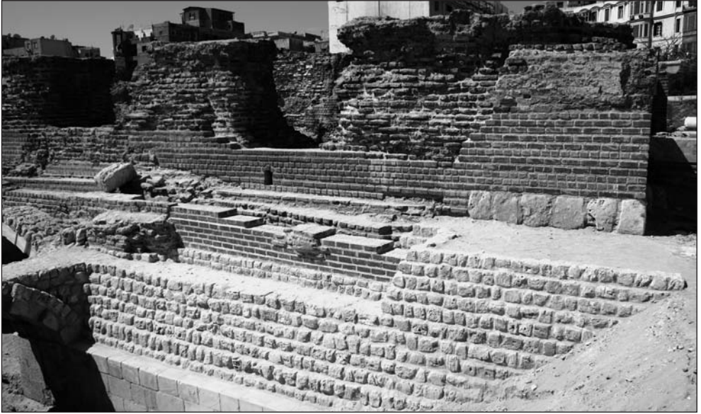
Fig. 14. Restored channel in the southeastern corner of the bath (Photo A. Pisarzewski)
