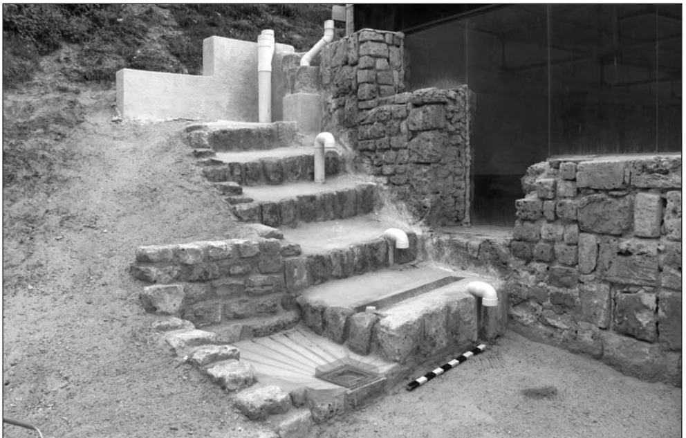
Fig. 11. Redesigned drainage system, plan and section (opposite page) and view of the southeastern corner of the shelter with the new drainage in place (top) (Drawing Z. Nawrot, M. Polak; photo G. Majcherek)
