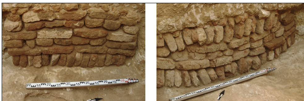
Fig. 5. Brick bonding in the blocking walls of chambers: left, main chamber (1) and right, chamber 3
