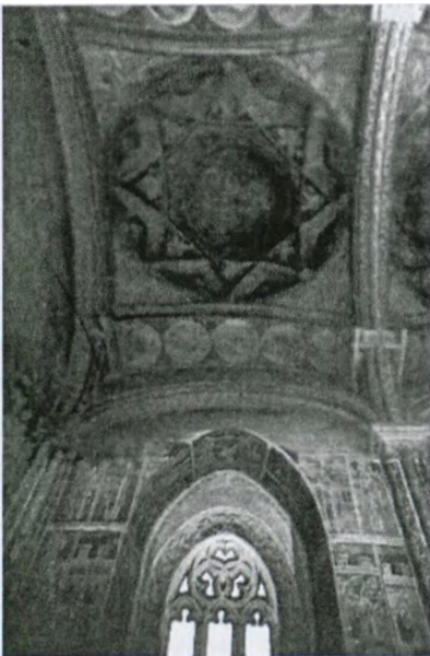
Fig. 6. Similar system of 'stepped arches' supporting a cupola: up, Lviv, Three Hierarchs Chapel, 1591; down, Moldavia, Probota church, narthex, 1530
