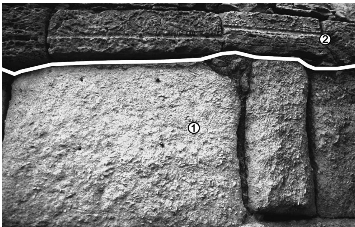
Fig. 7. Thickening of Turret XVI (R. Karasiewicz-Szczypiorski). 1 – blocks of Inkerman stone; 2 – fragments of secondarily used architectural details.
