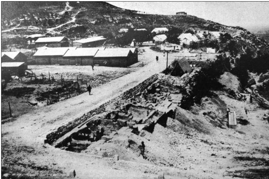
Fig. 3. Cyrene, military storerooms in the area of sanctuary of Apollo (on the left), access road partly covering Roman baths (on the right) in 1913 (after E. GHISLANZONI, Gli scavi delle terme romane a Cirene , “Notiziario Archeologico del Ministero delle Colonie” 2, 1916, 8).
