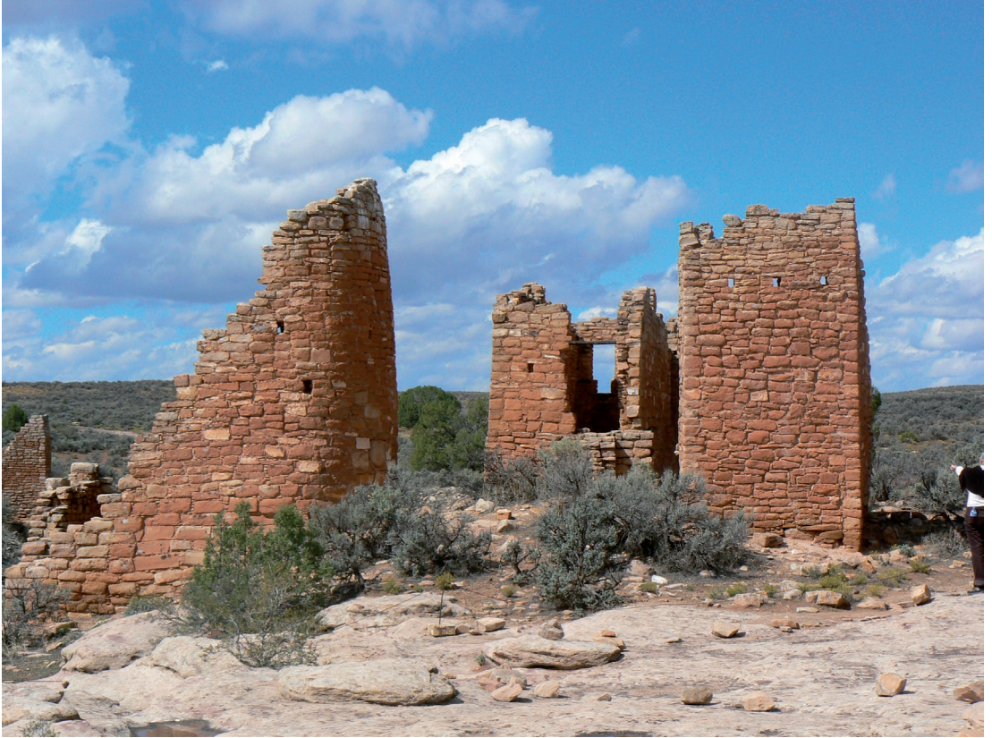
Fig. 36. Towers in Hovenweep National Monument (Southeastern Utah), photo by R. Palonka.
