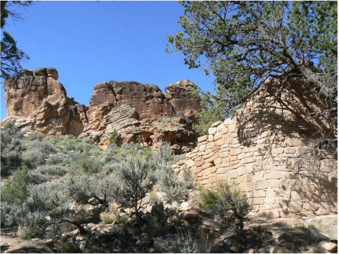
Fig. 7. Castle Rock Pueblo: Structure 404/409 (tower) with loophole in east wall. In the foreground the north face of the butte. Photo by R. Palonka.
