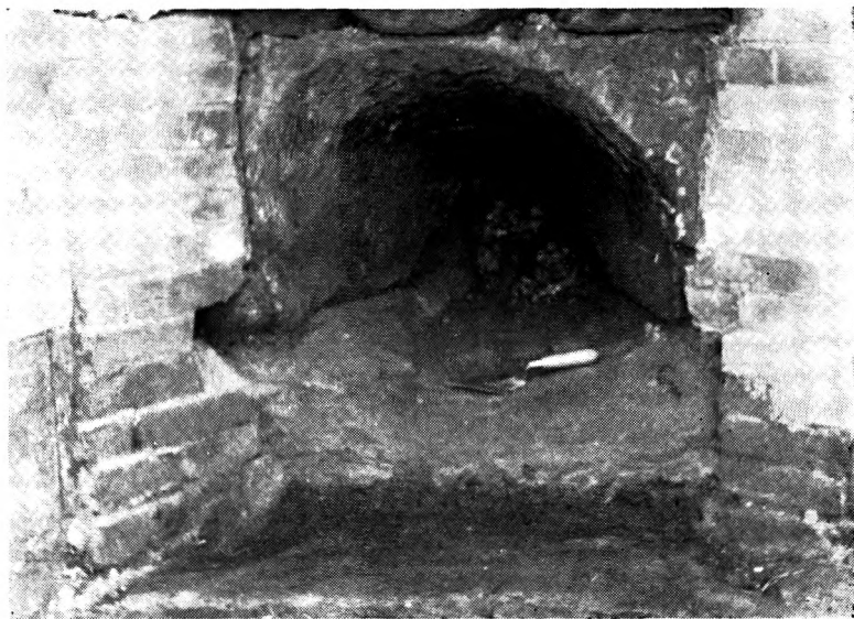
Fig. 13. Tuyere of furnace at Melbourne, Derbyshire (1725—1780)
