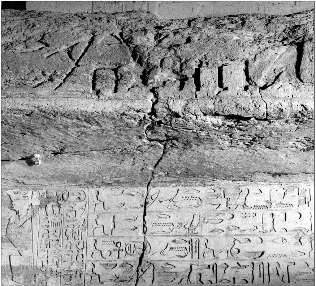
Fig. 1. Façade of the funerary chapel of vizier Meref-nebef. Re-inserted fragments of the "outer architrave" (Photo J. Śliwa)
