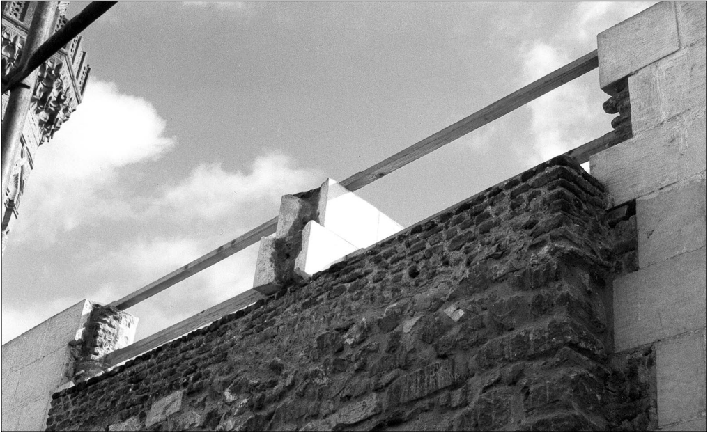
Fig. 1. Khanqab. Upper part of the northwestern elevation crowned with a safety balustrade between newly reconstructed Mamluk-like sections (Photo J.J. Kania)
