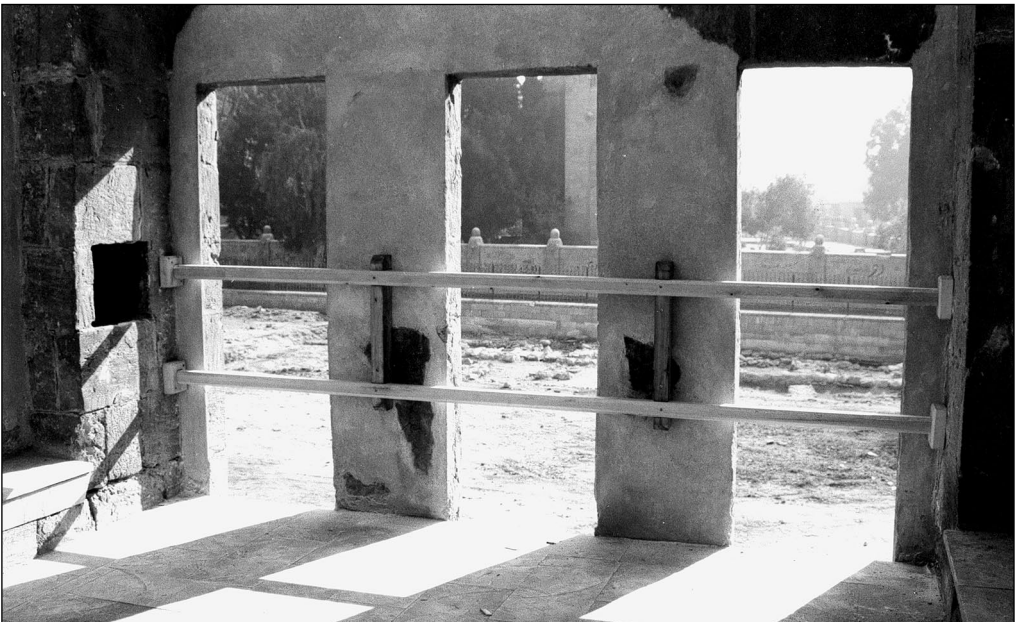
Fig. 2. Khanqab. Upper floor of the southeastern outer wall. Safety balustrade viewed from the interior (Photo J.J. Kania)
