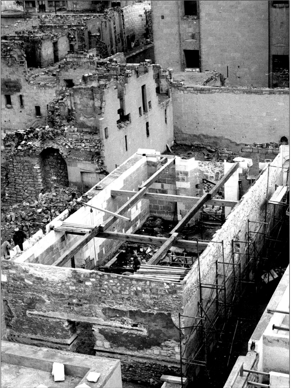
Fig. 8. Tabuna. Eastern building. The main structural timbers. State during roofing works (Photo J.J. Kania)
