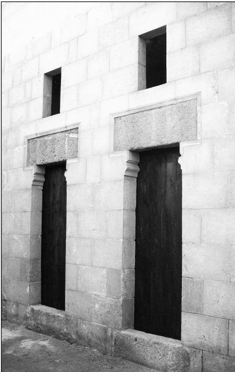
Fig. 3. Khanqah. Lower part of the restored northwestern elevation. Two entrances leading to the separate residential units. State after mounting the wooden shutters (Photo J.J. Kania)
