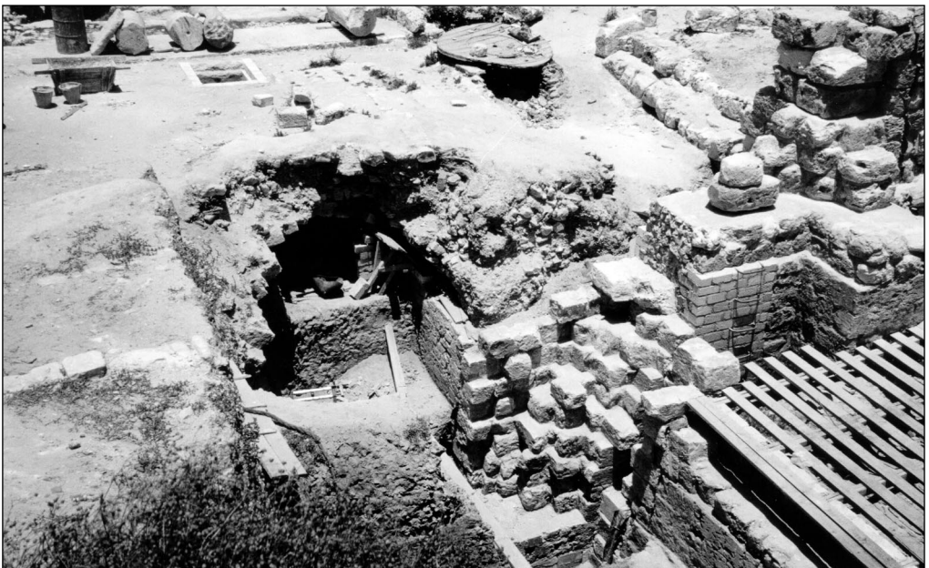
Fig. 4. Roman baths. Western section of the southern outer wall after anastylosis (Photo W. Kořataj)
