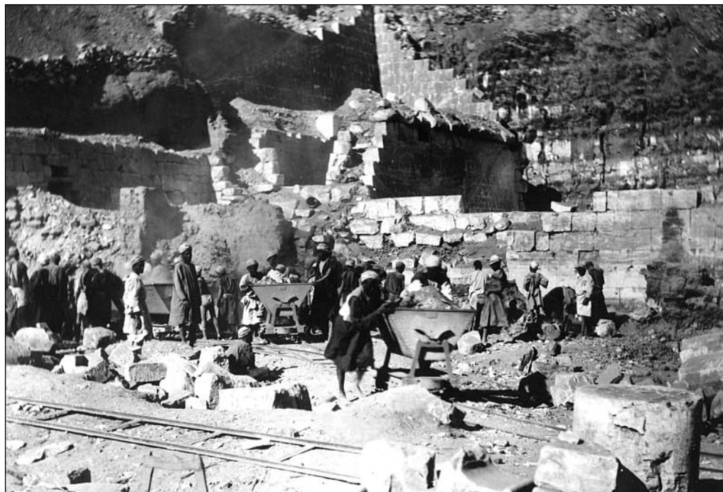
Fig. 9. Excavations of the Egypt Exploration Fund at the northern end of the Upper Terrace of the Hatshepsut Temple. Unearthed walls of the North Chapel of Amun-Re (Photo H. Carter, Courtesy of the Egypt Exploration Society, London)
