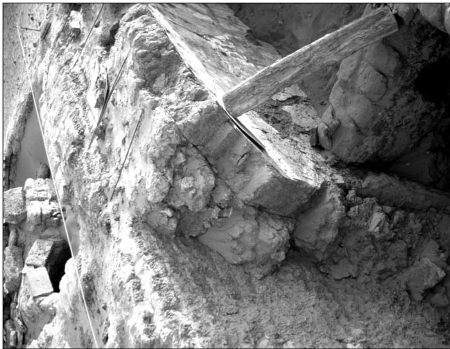
*Fig. 13. Destroyed vault in room 6 over the entrance to room 7 and the Terminal Christian wall supporting the vault (Photo W. Chmiel)*
