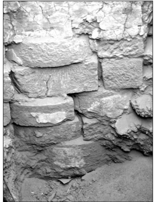
Fig. 5. Foundation beneath the northeastern pier of the Lower Church (Photo B. Żurawski)
