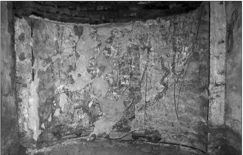
Fig. 5. Chapel 5. Earlier painting after cleaning and infilling of the gaps (Photo C. Calaforra-Rzepka)
