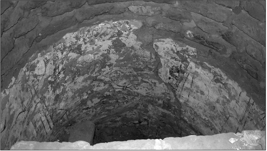
Fig. 6. Chapel 6. During the dismantling of the blocking wall: later painting with partial facing and the earlier painting uncovered (Photo C. Calaforra-Rzepka)
