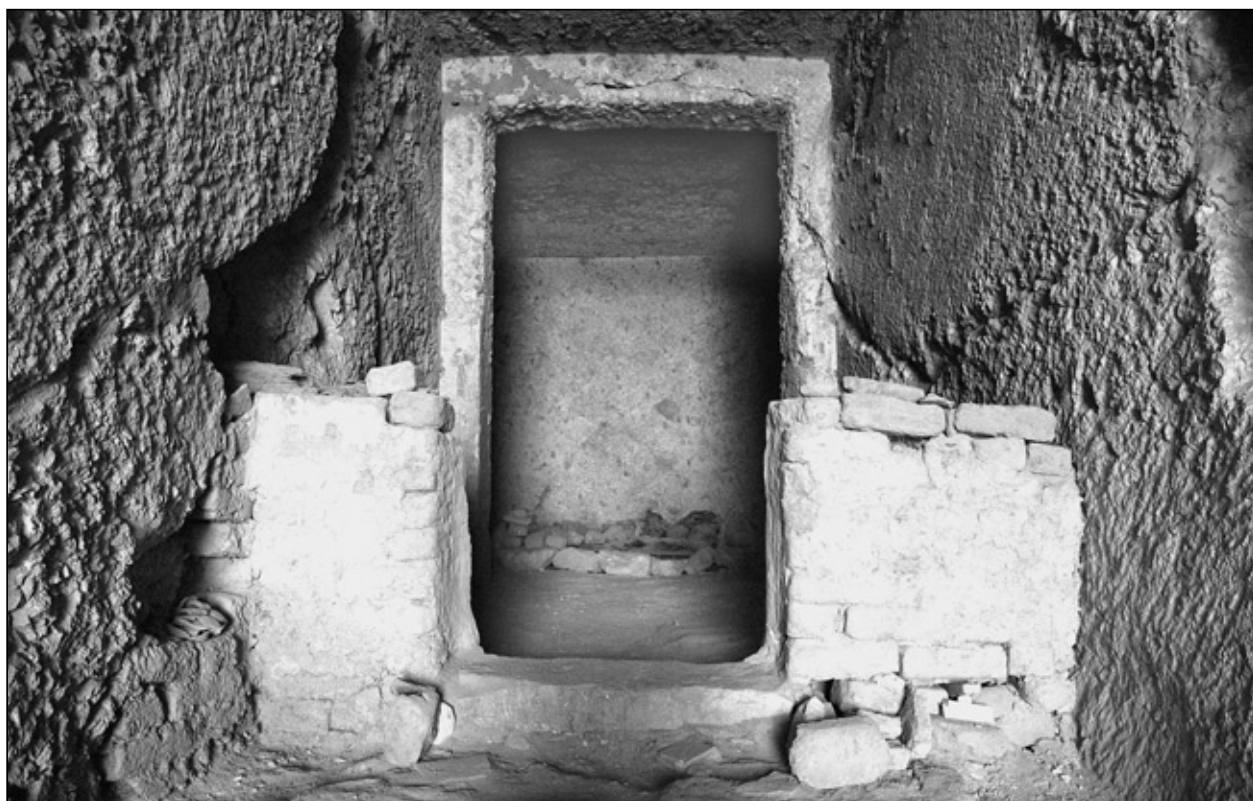
Fig. 2. Mud-brick wall separating the inner room from the front part of the hermitage (Photo T. Górecki)
