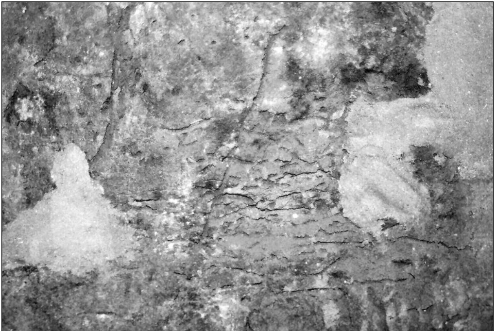
Fig. 4. Face of mural from the Lower Church (after application of putties and preliminary reinforcing of the plaster structure), demonstrating a full gamut of damages: termite tunnels, white spots of salt crystallization – chiefly gypsum, black fungi (?) colonies (Photo D. Moryto-Naumiuk)
