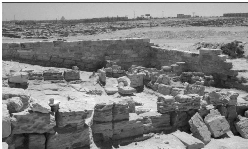
Fig. 2. House H1. Reconstructed perimeter wall in the southeastern part of the structure, state in 2006 (Photo S. Medeksza)
