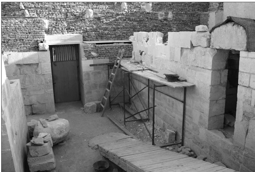
Fig. 1. View of the courtyard in the Royal Mortuary Cult Complex during the dismantling of the east wall in 2007 (Photo O. Białostocka)
