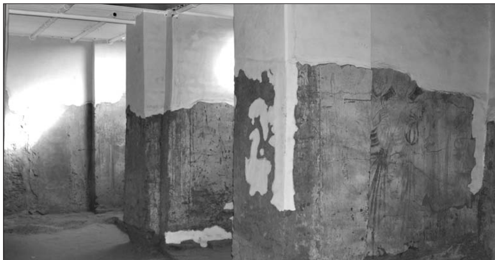
Fig. 5. Interior of the Raphaelion with plastered upper section of the walls in the northern part of the khurus (Photo B. Żurawski)
