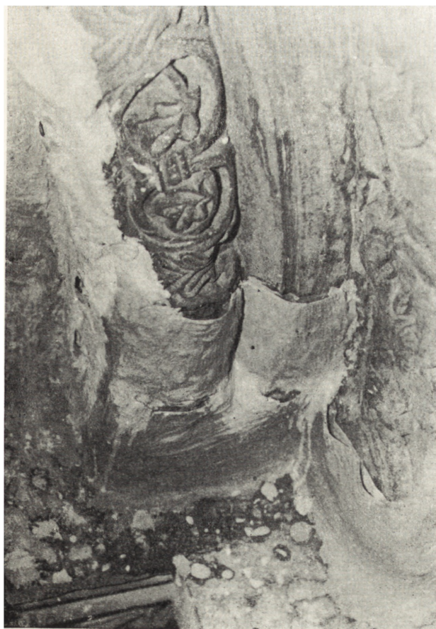
7 a—e. Doorway from Ołbin — Consecutive stages of pocket laying on the doorway surface
