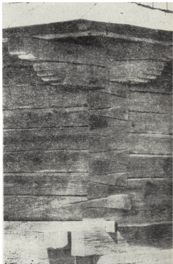
4. Fragments of structural carcasses with decorative beams: (a) at Hulcze, 1869 (a sill bearing the church „erection record”), (b) at Sulimów, 1867 (a sill), (c) at Budynin, 1887
