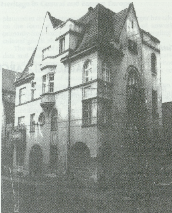
4. Lwów, ul. Puszkina (d. Potockiego) 68. Dom mieszkalny, 1913 r. 4. Lvov, 68 Pushkin Street (formerly Potocki Street). Residential building 1913
