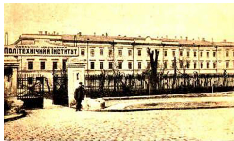
Fig. 8. Saban barracks: the first building of the Odessa Polytechnic Institute (source: “Poželaem zvezde politeha imenami vse ârče goret...”: temat ukaz lit posviashch 100-letiu ONPU, Odessa 2018)
