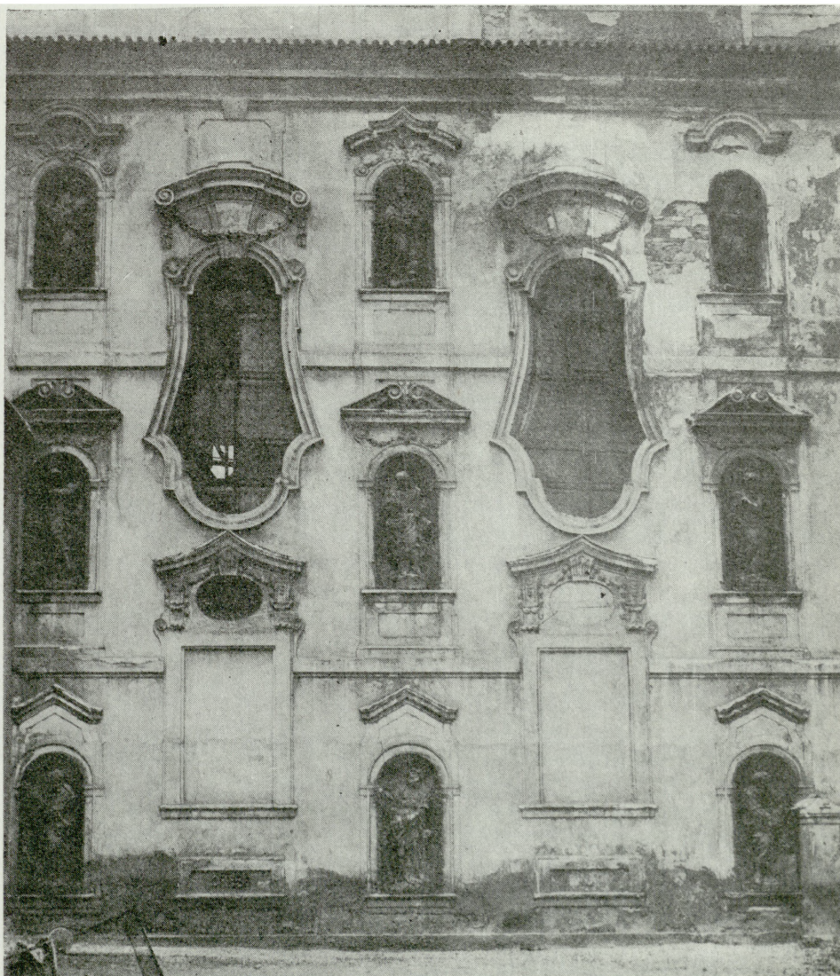
18. North elevation of the Church, its middle part
