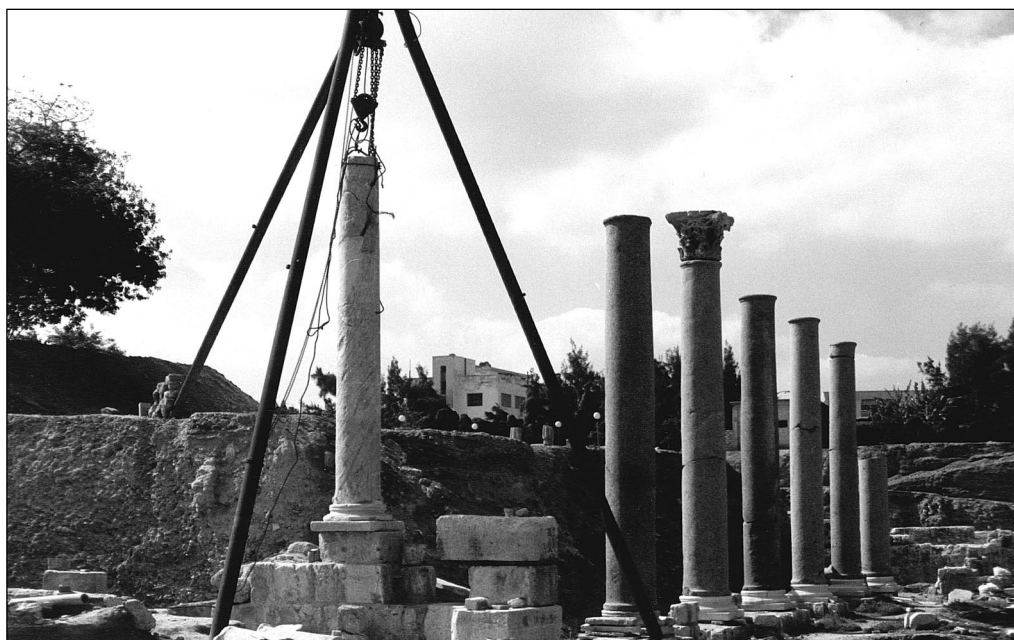
Fig. 6. Anastylosis of a marble column from the southern gymnasium (Photo W. Kołtątaj)
