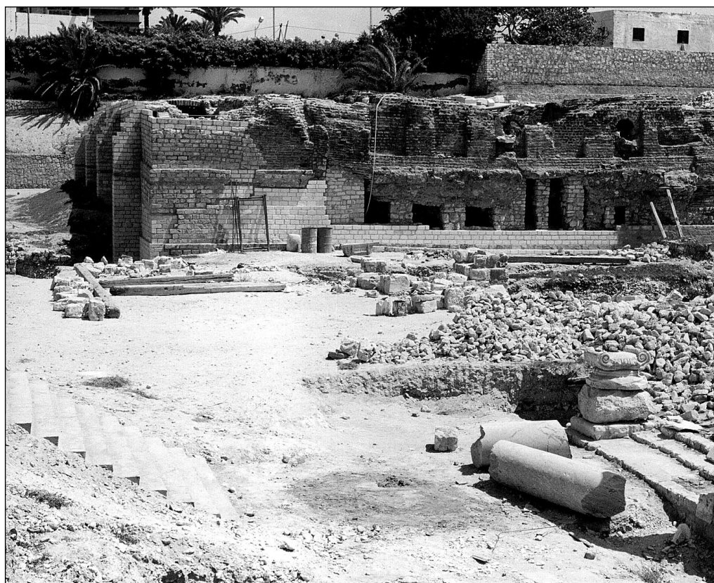
Fig. 7. Cistern. The northern facade during reconstruction works (Photo W. Kolqataj)
