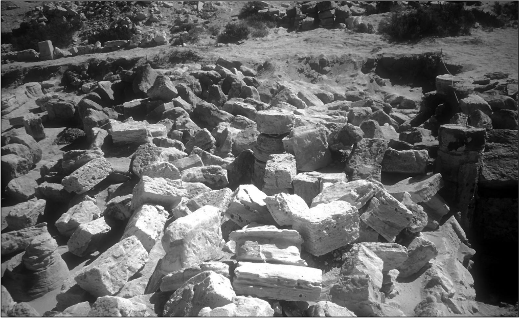
Fig. 16. Town center. Collapsed wall in southeastern corner of main square, view from the northwest (Photo W.A. Daszewski)
