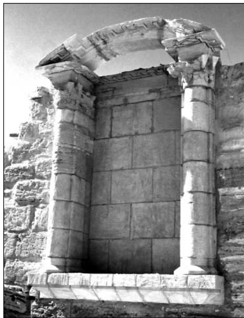
Fig. 4b. Wall niche from hall H 21N. View following anastylosis in 2003 (Photo S. Medeksza)
