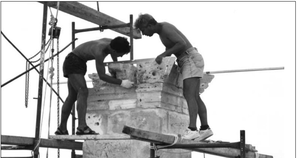
Fig. 7. Anastylosis of the capital on top of pillar tomb T 1K (Photo S. Medeksza)
