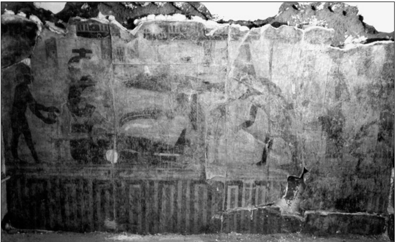
Fig. 3. West wall of the sanctuary after remounting of the mural paintings. Condition in 2005 before removal of the facing (Photo R. Rogal)
